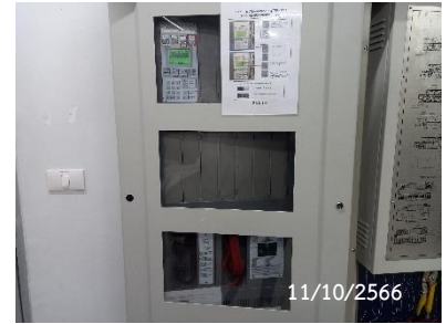
Fire Alarm Control Panel
