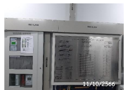
Graphic Annunciator Fire Alarm System
