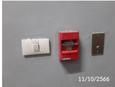
Fire Alarm Manual Station
